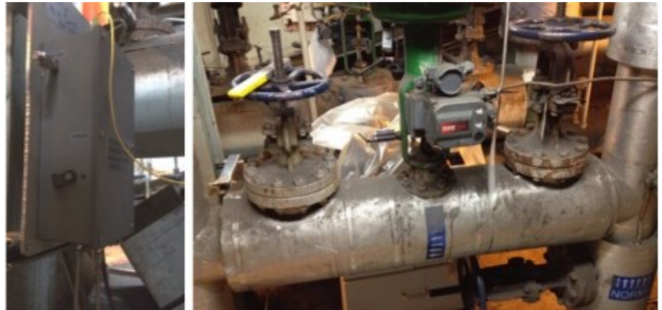
Figure 1: Photographs of installation of sensor (left) in PSU Steam Plant to measure pressure across the boiler feedwater valve (right).
