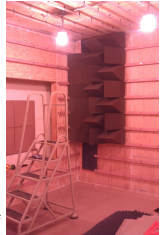
Interior shot of the hemi anechoic chamber during construction.
